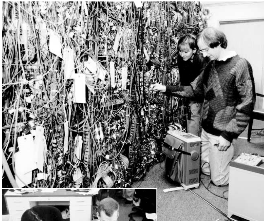
Lucy deBarbaro (above), a postdoc from Northwestern University, and Howard Budd, a senior research associate, fix a bad logic unit in the trigger room.
