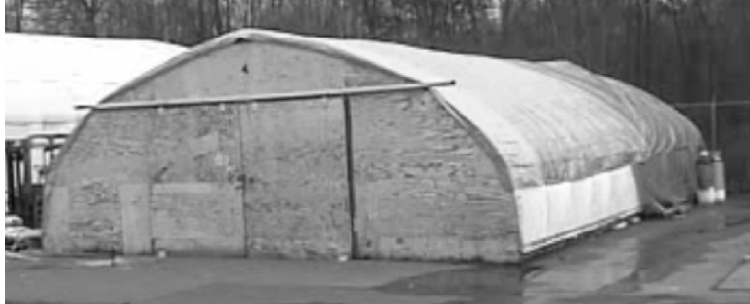
Figure 2.2 Remote Manufacturing Demonstration Building Exterior
