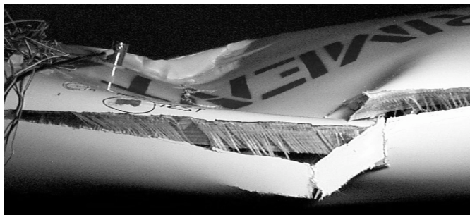
Figure 1.7 Photograph of the ERS-100 Panel Buckling Location
