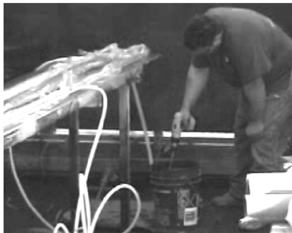
Figure 2.15 Mixing Resin Prior to Infusion
