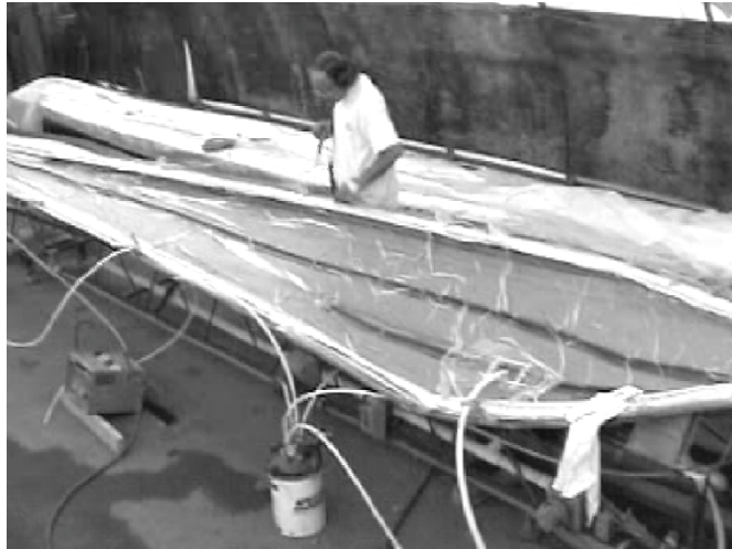
Figure 2.14 Inspecting for Vacuum Leaks Before Skin Infusion
