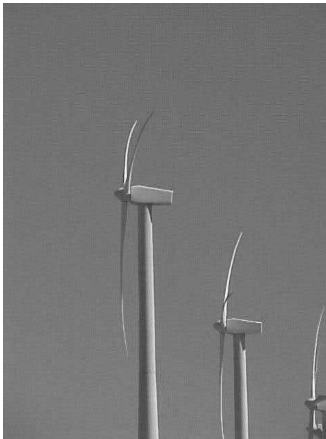
Figure 9 Vestas V-47 Rotors under Aerodynamic Loading
