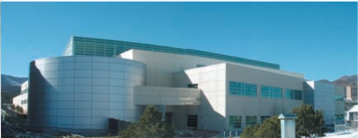
Figure 21. The new Strategic Computing Complex (SCC) — Nicholas C. Metropolis Center for Modeling and Simulation at Los Alamos National Laboratory.
