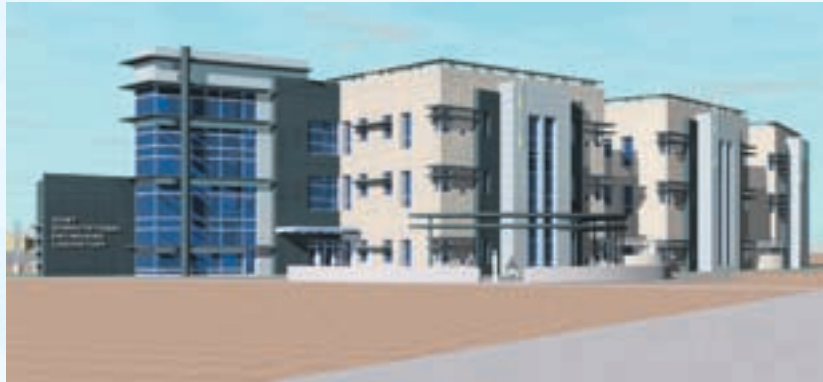
Figure 23. The JCEL at Sandia National Laboratories in Albuquerque, NM.
