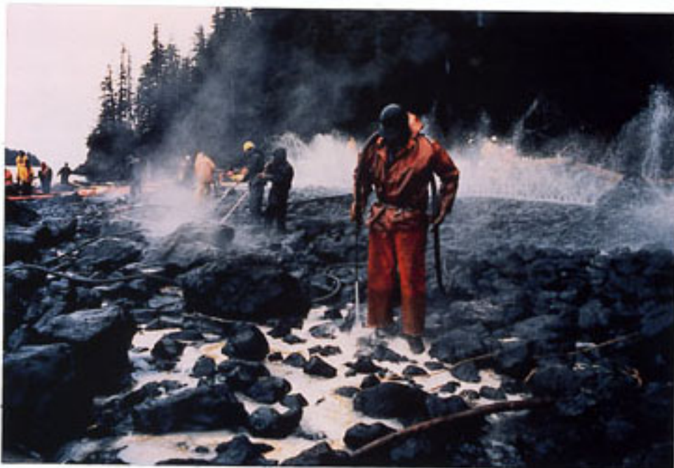
Plate 19. Shoreline treatment using a chemical shoreline cleaner after the Exxon Valdez oil spill in Prince William Sound, Alaska (NOAA/HAZMAT photo)
