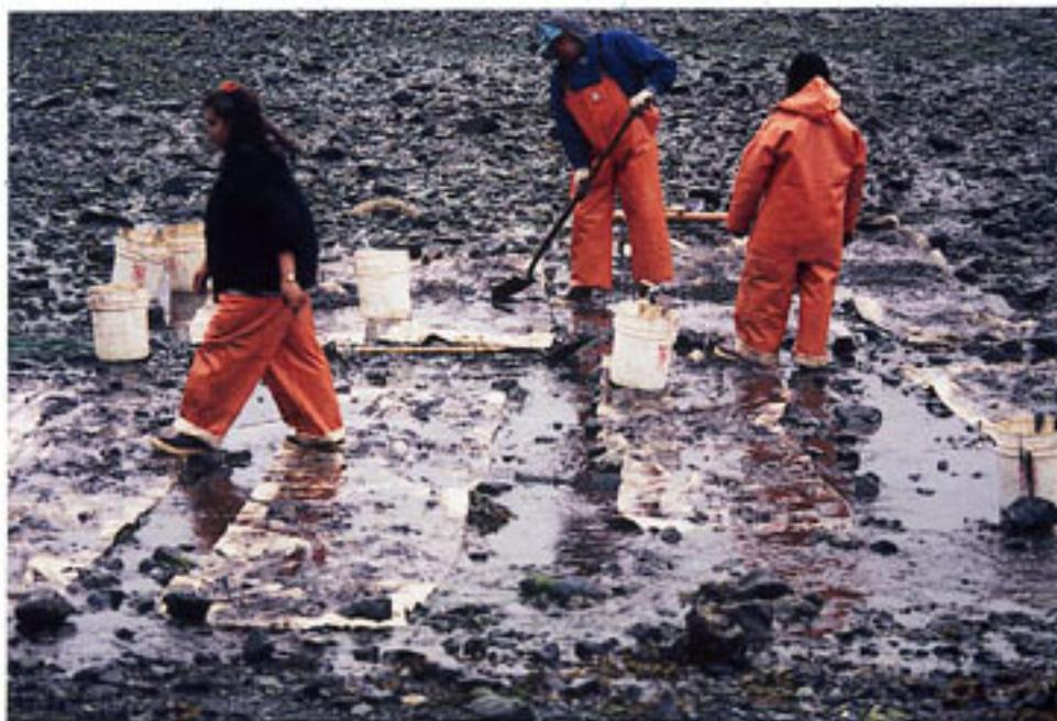
Plate 20. 1994 mussel bed cleanup activity in Prince William Sound, Alaska. Oiled sediments have been moved to lower intertidal zone for tidal flushing of residual oil (Photo by A. Mearns, NOAA)
