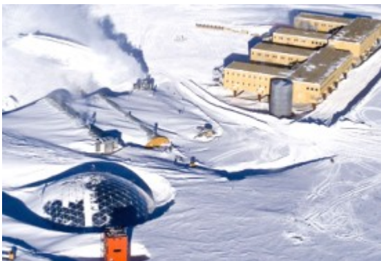
This aerial photo from October of 2005 shows the new South Pole Station (without its final outer layers) in the upper right portion of the frame. The old station is the geodesic dome at the lower left. Credit: Scot Jackson, NSF.
