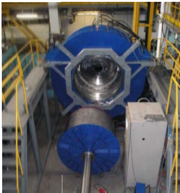
Figure 3.10. Back view (ground plane side) of the voltage adder with the cathode electrode outside.
