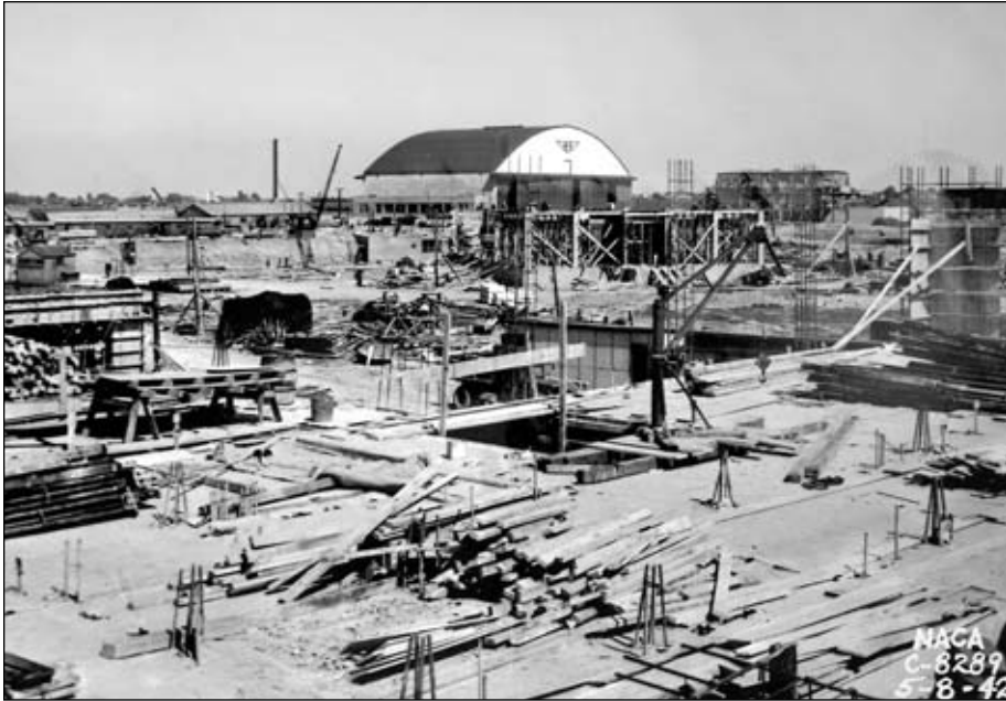
Figure 2-2. Construction begins for the AERL, 8 May 1942. (NACA C-8289)
