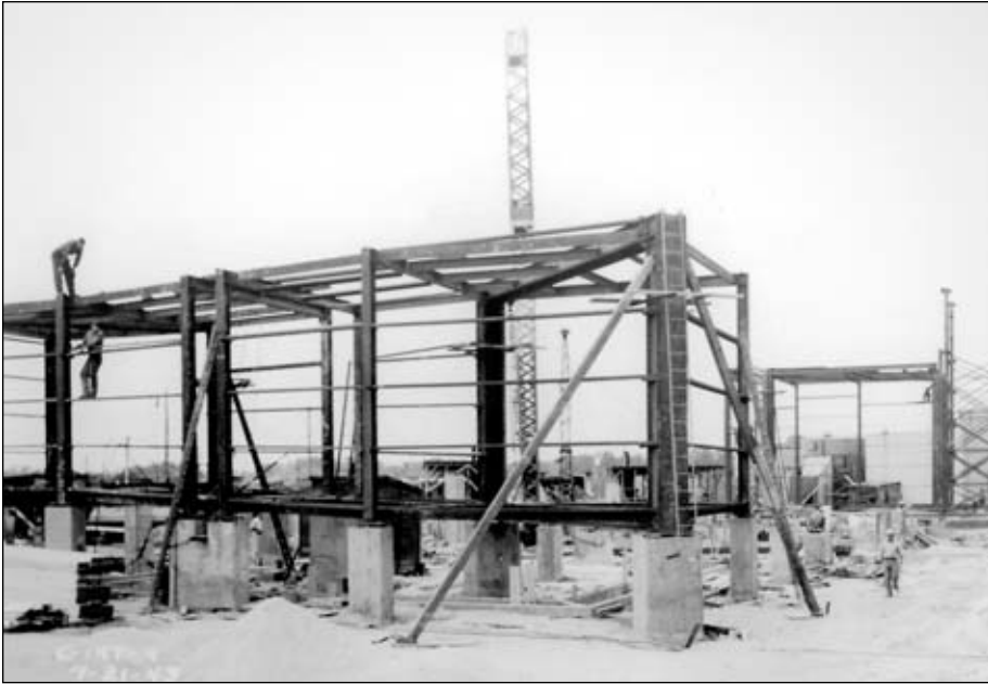
Figure 2-3. Shell framing for the Icing Research Tunnel, with Altitude Wing Tunnel in background, 21 July 1943. (NACA C-IRT-4)
