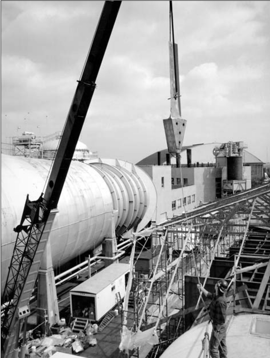
Figure 7-3. IRT renovation, 1993. (NASA C-93-7170)
