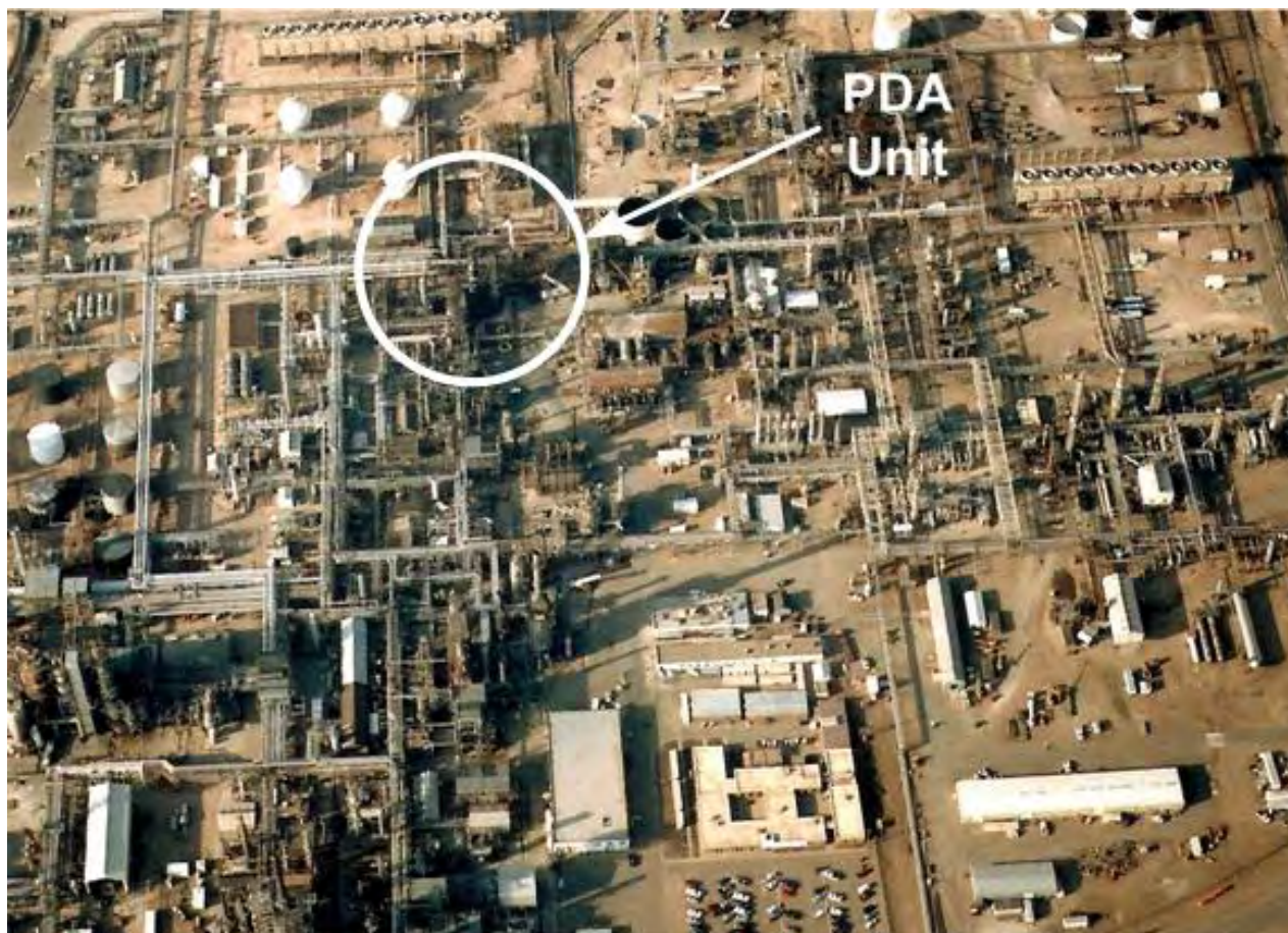
Figure 1. PDA unit location in the McKee Refinery
