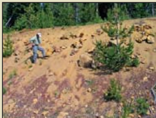
Figure 5.49 – When cut and fill slopes reach their angle of repose, non-cohesive soils move downslope at a continuous rate. The soil surface is constantly moving and never stable long enough for seeds to germinate and plants to become established. These slopes can remain barren for years. Soils that are high in sands and gravels are the most susceptible to dry ravel. In this picture, trees became established below rock outcrops, where the surface was protected from dry ravel.
