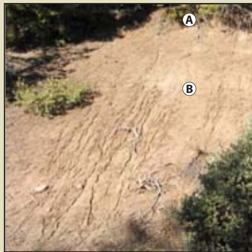
Figure 5.53 – Surface erosion increases with distance downslope. On this site, sheet erosion turns to rill erosion at point B. Mitigation that shortens slope lengths to less than the distance between A to B will reduce rill erosion.
