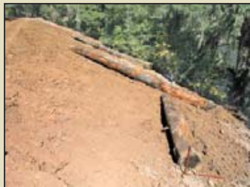
Figure 5.31 – Placement of large wood adds long-term organic matter while creating microsites for planting seedlings. Large wood can also slow runoff and detain sediments from surface soil erosion.
