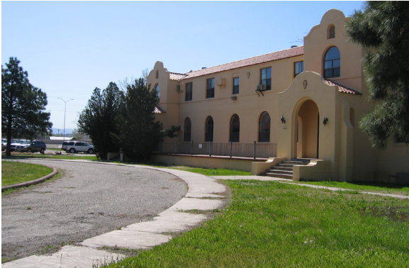
Images showing street conditions, the new addition to the Indian Pueblo Cultural Center, and the only remaining building from the Albuquerque Indian School.
