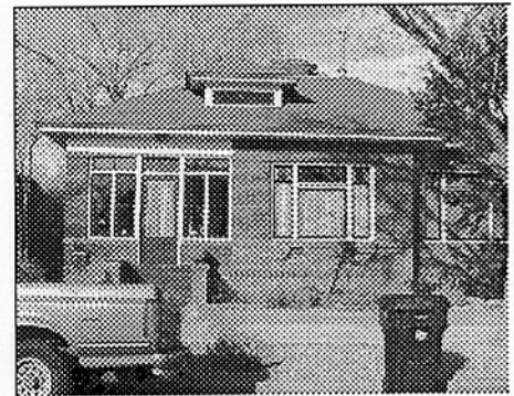
The front porch (left side of photo) at 1015 Roma NW has been enclosed with glass set in wood framing. The porch enclosure's design is appropriate in its materials and similarity to the pattern of the house's original windows.
