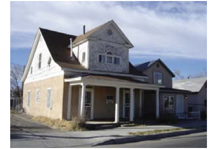
917 3rd Street SW, built around 1898
