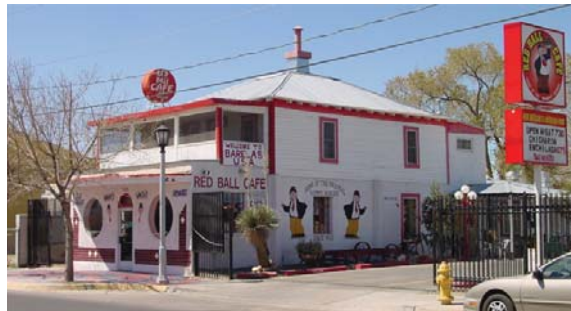
The Red Ball Café This neighborhood fixture was renovated in 1998, and remains a vibrant gathering place in Barelás.
