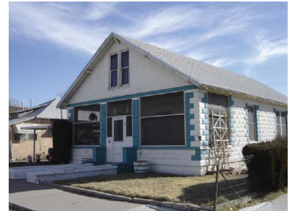
524 Iron SW, built about 1912
