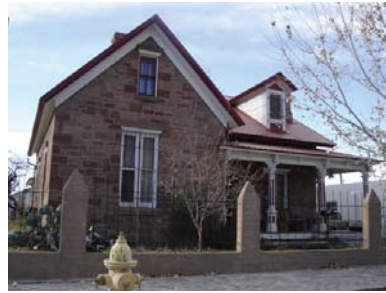
1023 2nd Street SW - Superintendent's House, Atlantic & Pacific Railroad - built 1881 and listed
