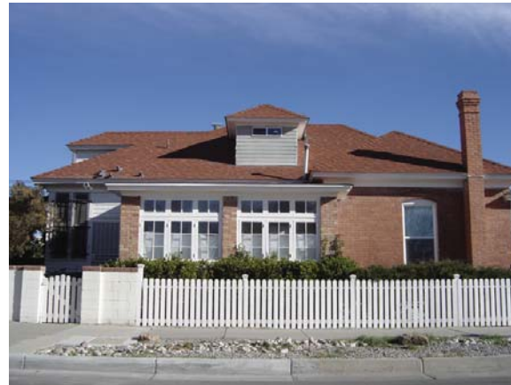
523 Iron SW, built about 1908
