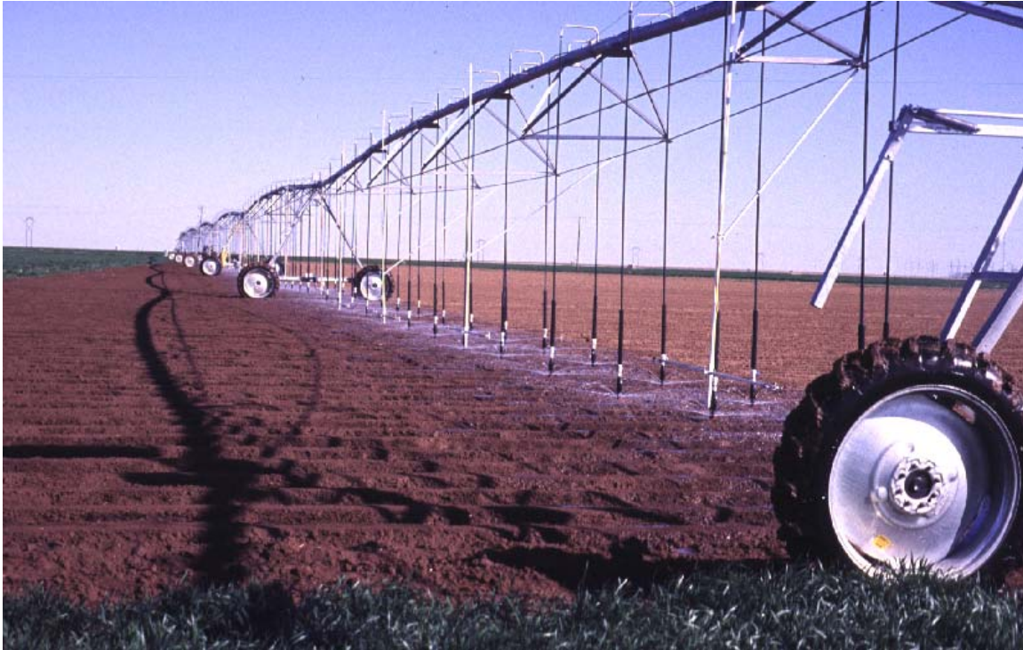
Figure 2. Typical example of a LESA system with spray heads on drops spaced 5 ft (1.5 m) apart).
