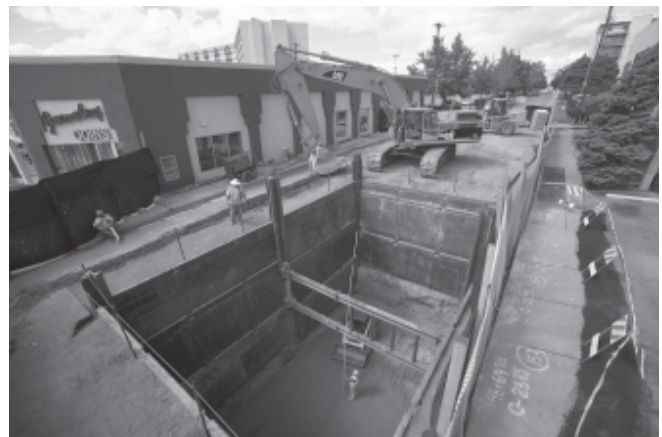
Pipeline Being Installed
