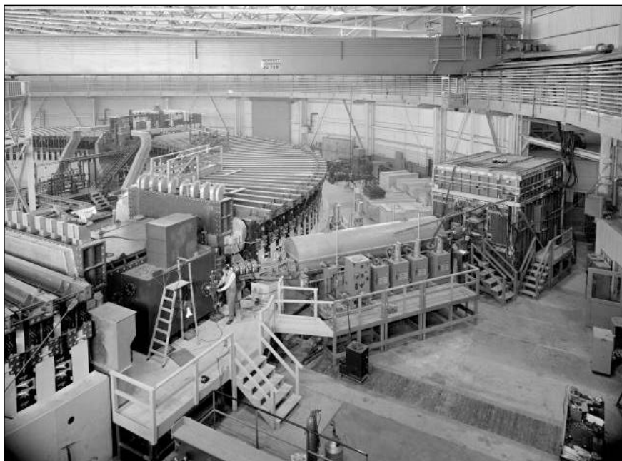
This file photo shows the Cockcroft-Walton accelerator, right, that fed protons into an Alvarez linear accelerator, center, for injection into the Bevatron accelerator at Lawrence Berkeley National Laboratory. The Bevatron was decommissioned seven years ago, but some of its steel plates will be used as shielding in a new spectrometer at the Los Alamos Neutron Science Center.
