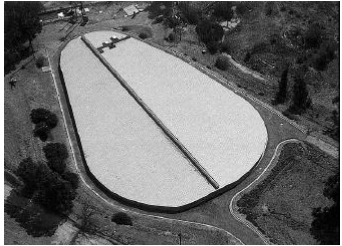
Covered finished water reservoir Source: Los Angeles Department of Water and Power (LADWP), 1988
