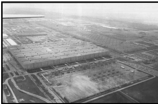
Figure 2: Portsmouth Gaseous Diffusion Plant
