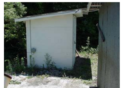
USGS 02337040 SWEETWATER CREEK AT WATER INTAKES, NEAR AUSTELL, GA
