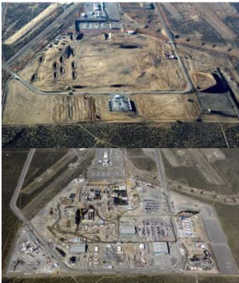
PNNL's S&T is supporting resolution of key technical issues within the WTP flow sheet and process design. Progress toward bringing the WTP online is evidenced by construction progress from January 2002 (top) and April 2003 (bottom).
