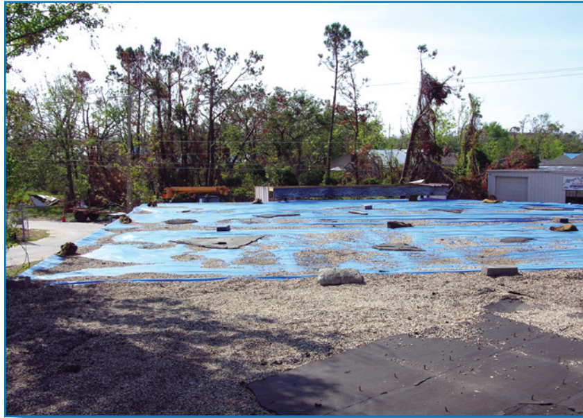
Figure 4-44: Roof damage at Hancock County EOC
