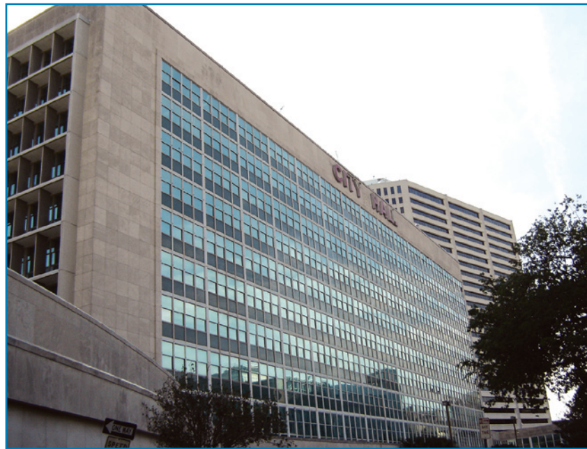
Figure 4-36: New Orleans EOC in the City Hall building
