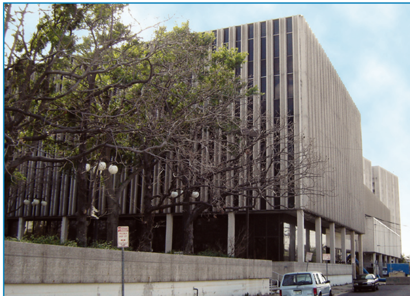
Figure 4-34: New Orleans Police Department Headquarters
