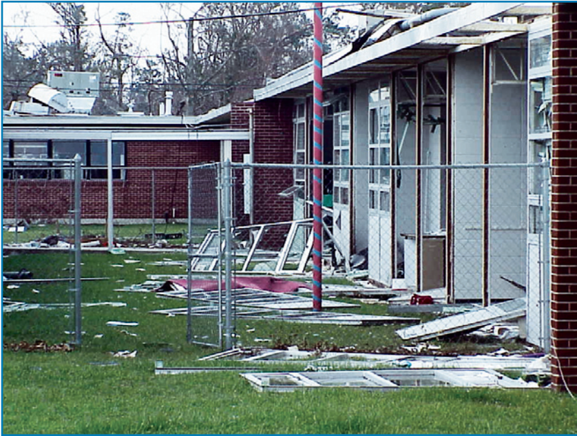
Figure 4-18: Pineville Elementary School shelter had to be evacuated when the floodwaters started to rise.
