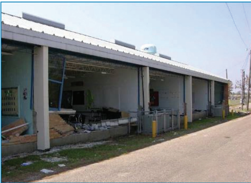
Figure 4-19: Exterior walls at Northbay Elementary School
