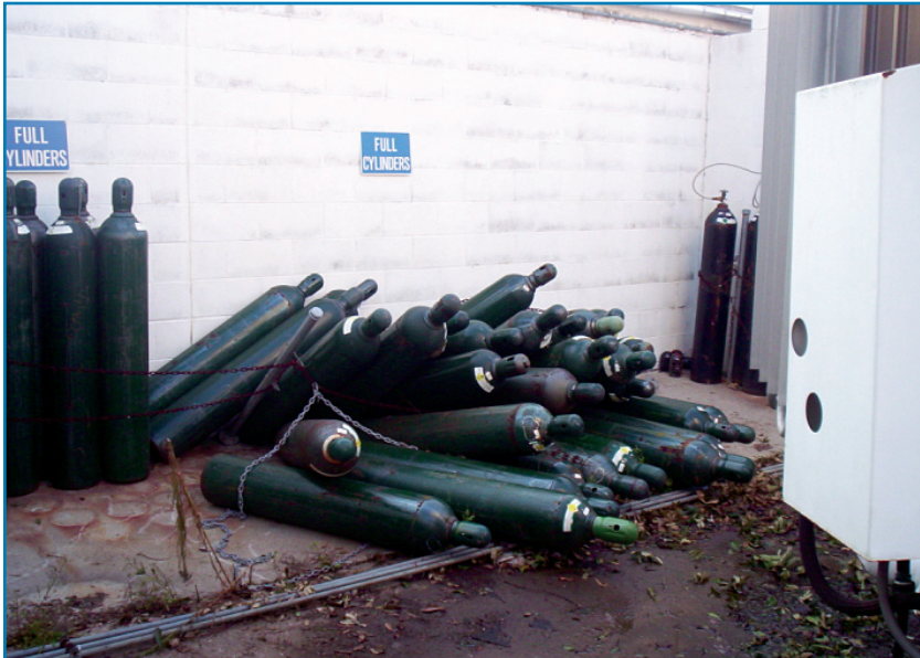
Figure 4-13: Oxygen supplies at Hancock Medical Center
