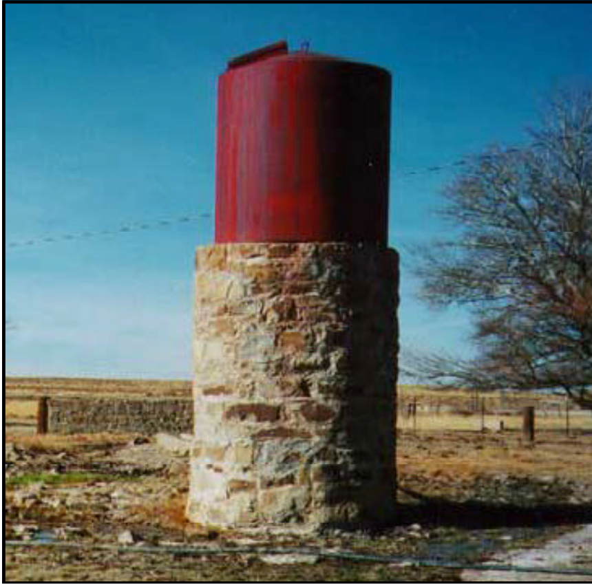
This 1,000-gallon storage tank is mounted on top of a stone structure to provide a pressure gradient.
