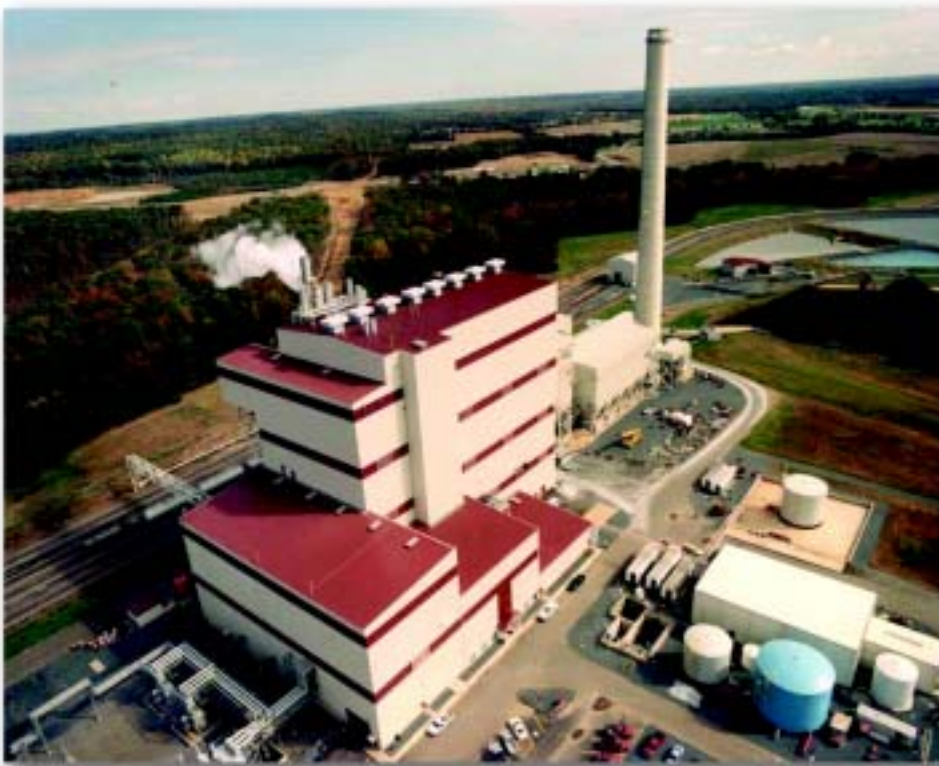
Mirant-Birchwood Power Facility in King George County, VA
