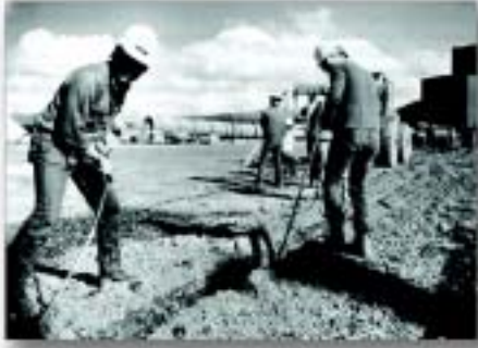
Laying Pipeline in Alaska
