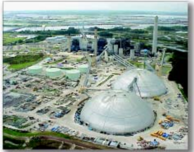
The JEA repowering project converted an existing oil/gas-fired steam plant to coal-fuel blends, and resulted in the largest circulating fluidized-bed unit in the world.
