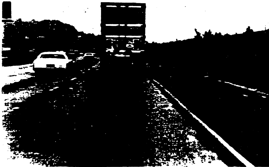
Photo 3 - A truck travelling near the edge of pavement. Note the pavement edge stripe location (12-ft PCC pavement slabs).
