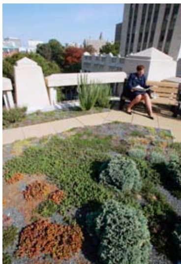
Green roofs, like this one in Atlanta, Georgia, are made of grasses and shrubbery and are designed to reduce energy use, filter pollutants from rainwater, and cool down cities during warm months.
