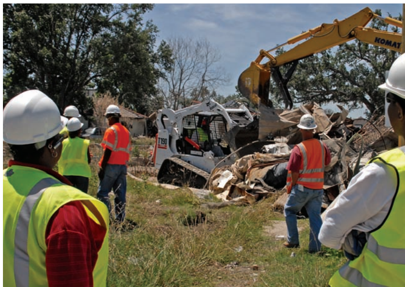
New Orleans, LA, May 11, 2006— Workers begin removing private property debris in the 9th Ward and putting it in curbside piles for removal to debris dump sites. FEMA is funding private property debris clean up. (Marvin Nauman/FEMA photo)
