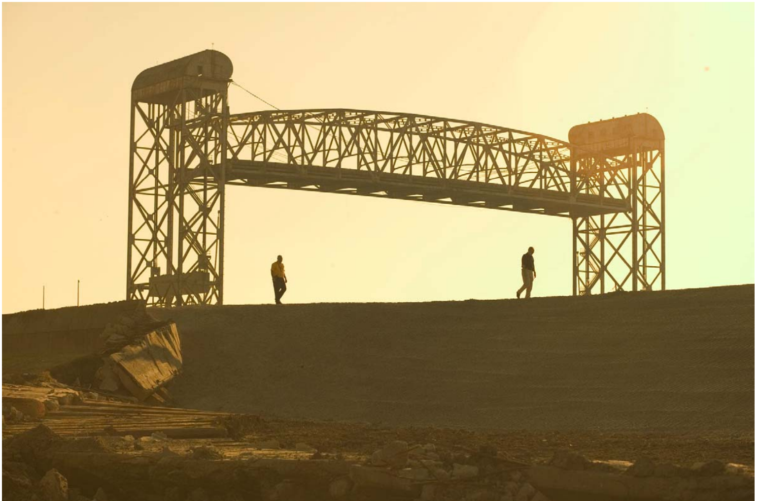
New Orleans, LA., October 17, 2005 -- Mike Chappell and Jim Gunnel from Department of Homeland Security look at the temporary levee built in the 9th Ward neighborhood following Hurricane Katrina. [Source: Andrea Booher/FEMA]
