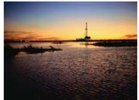
An oil and gas production facility co-existing safely with local flora and fauna in a sensitive Gulf Coast marshland.
