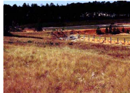
The range was restored by controlling storm water runoff and stabilizing slopes using diversions, sediment traps, and permanent vegetation.
