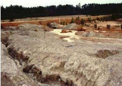
This range was constructed in the 1950s or 1960s before consideration was given to storm water management and erosion control.
