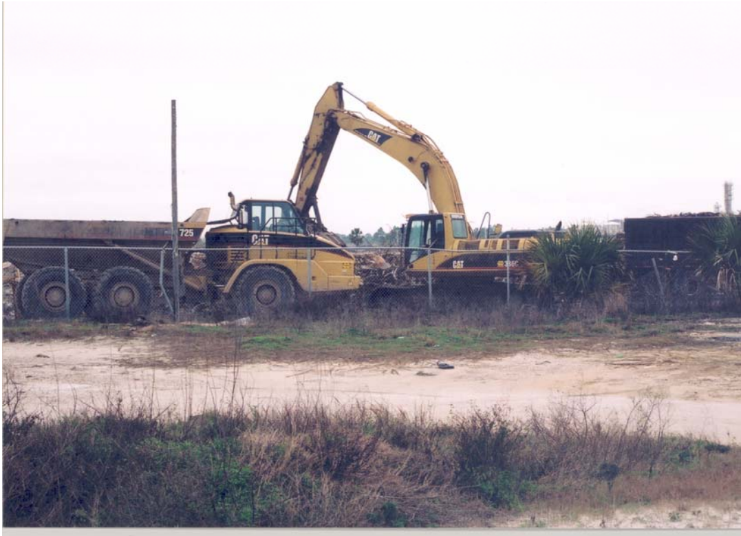
Photo 4: Bucket loader and dump truck, southern parcel.
