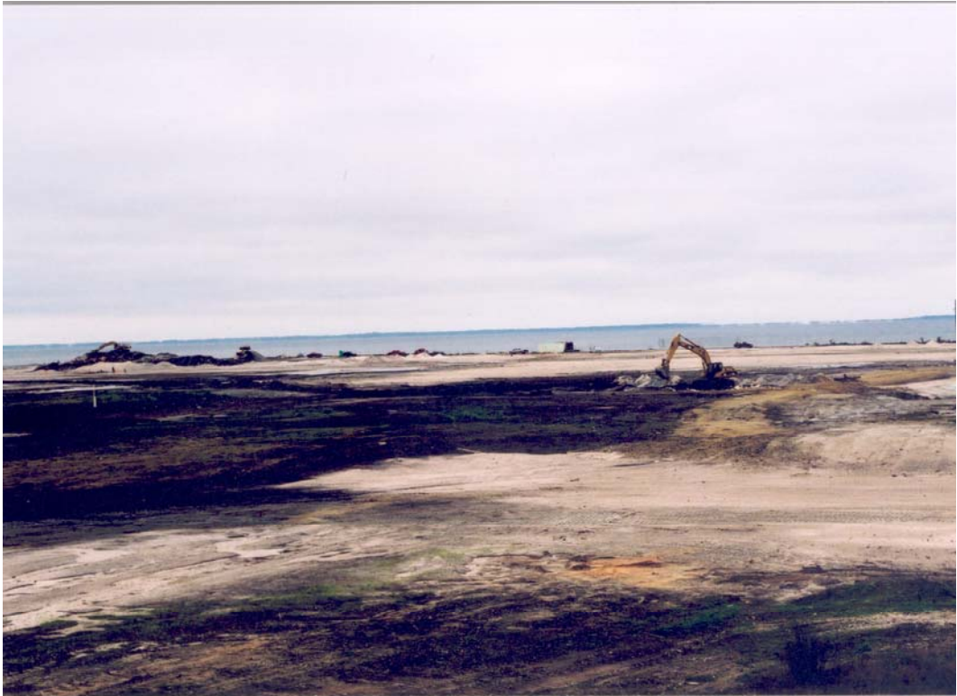
Photo 7: Soil capping operations on the southern parcel.
