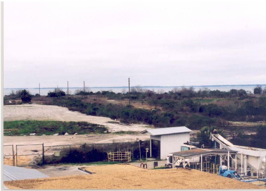
Photo 9: View to the northwest from the bridge, vegetated area forms the southern boundary with the northern part of the site.
