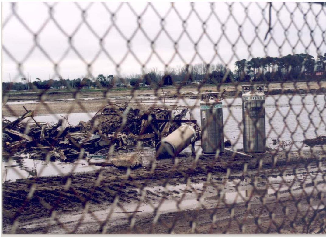
Photo 3: Metal debris and oxygen tanks on the southern parcel.
