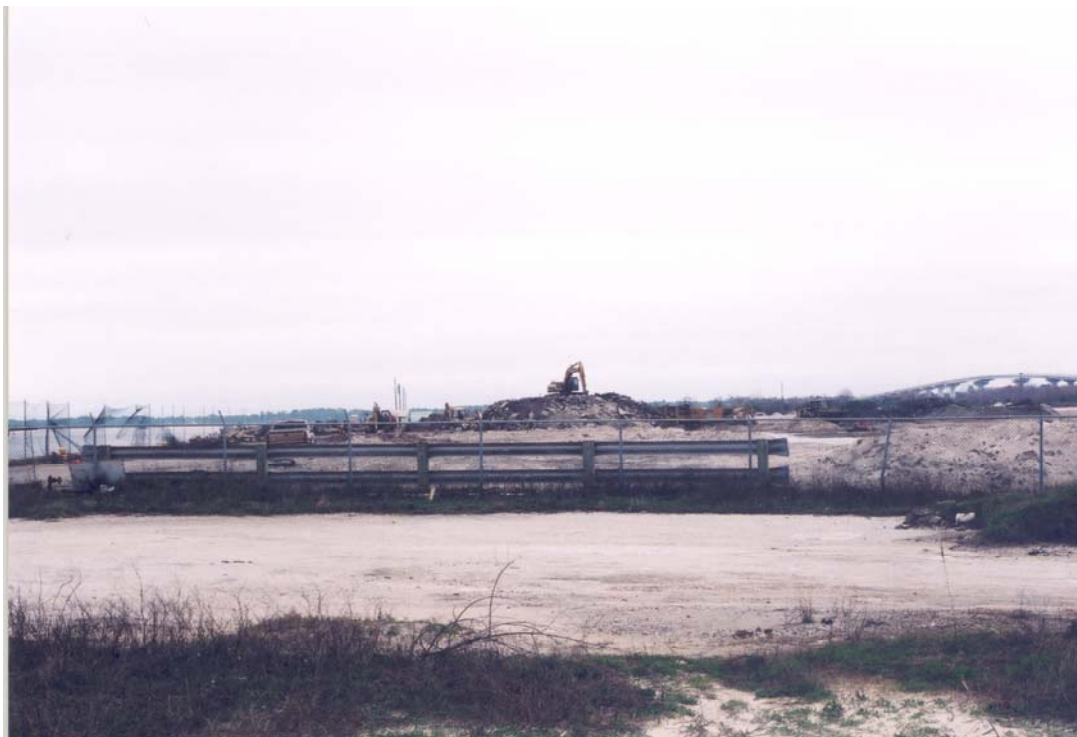
Photo 5: Rubble pile and removal equipment on the the southern parcel.
