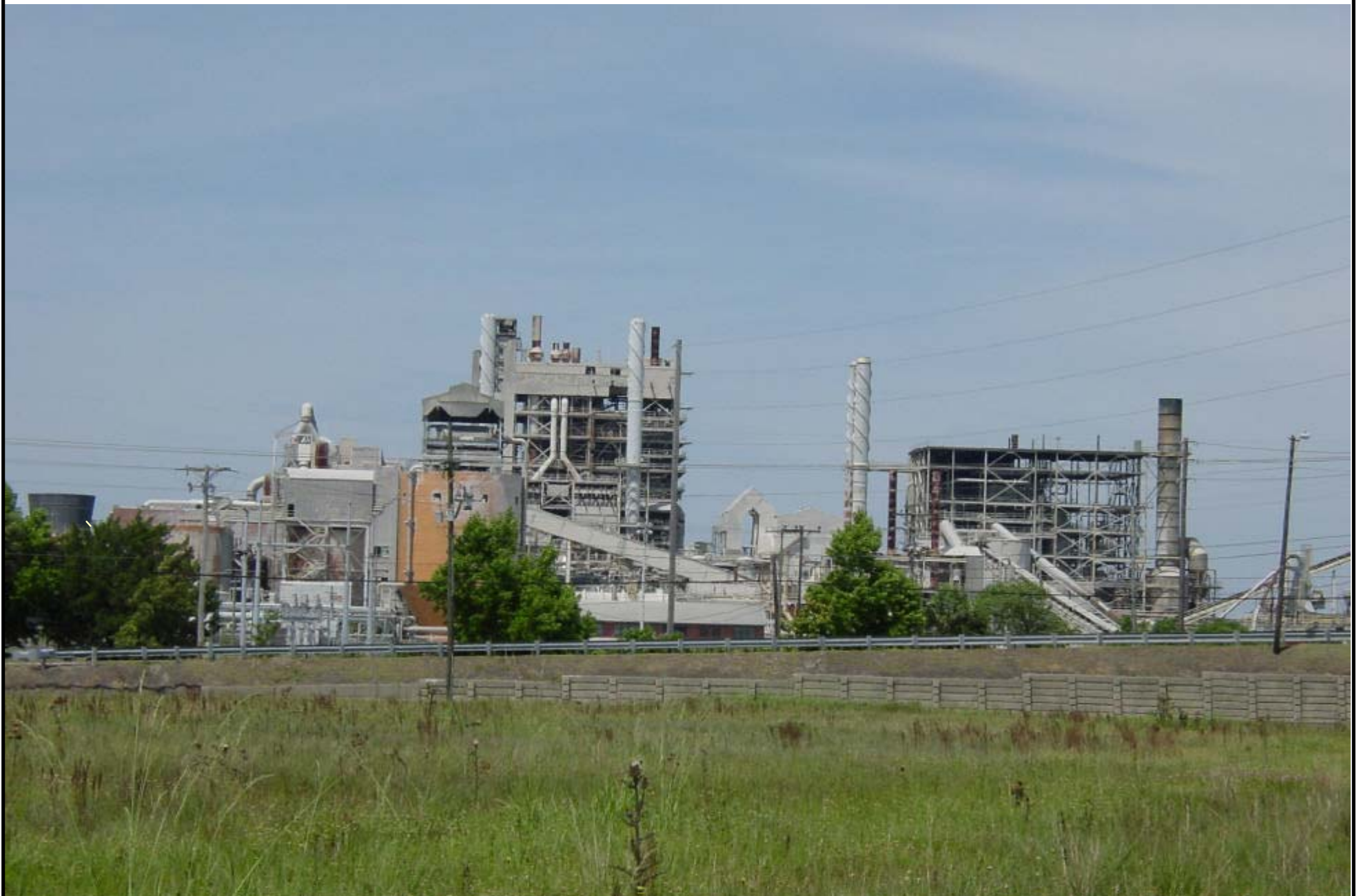
Photograph 1: Closed St. Joe Millworks former St. Joe Forest Products site Port St. Joe, Gulf County, Florida
