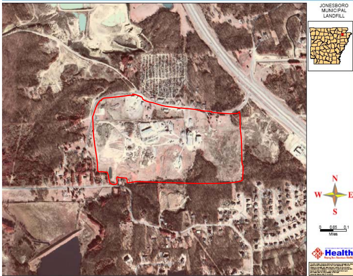
Figure 1. Jonesboro Municipal Landfill Aerial Photo
