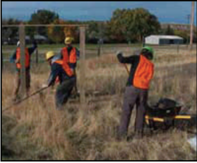
Photo of work crew installing New recreation area identification signs.
