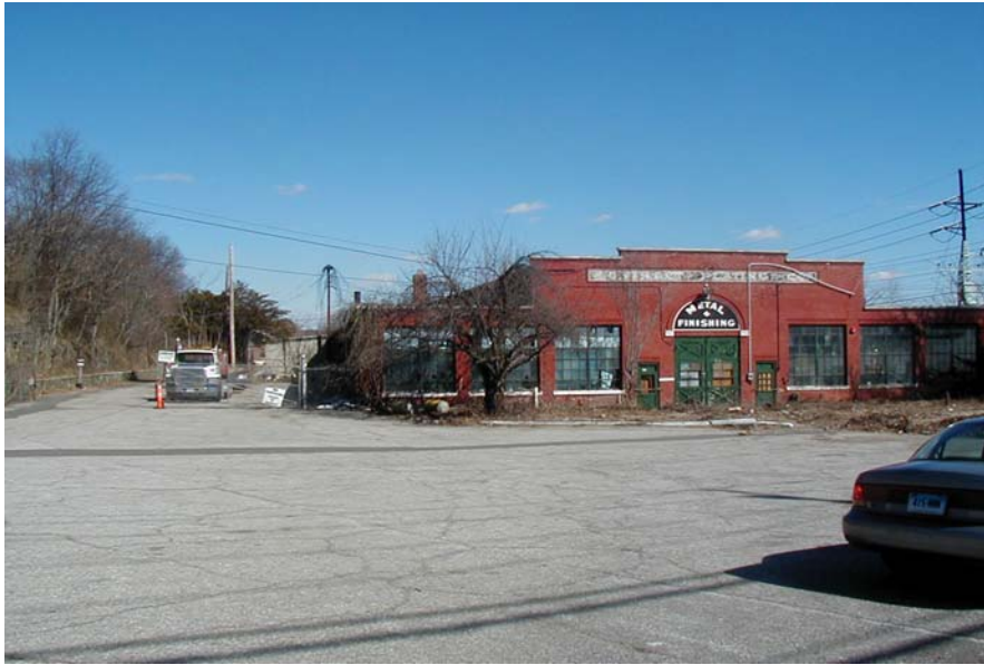
Front of Main Process Building
