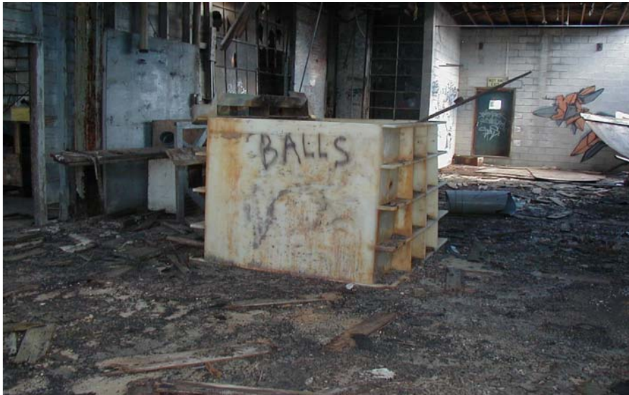
Interior of Main Process Building – Evidence of Trespassing
