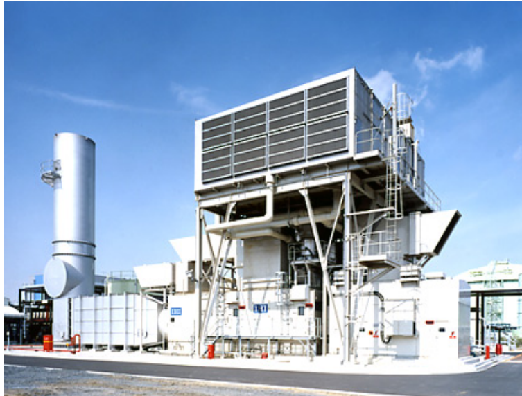
Figure 4. Typical simple cycle gas turbine power generator
