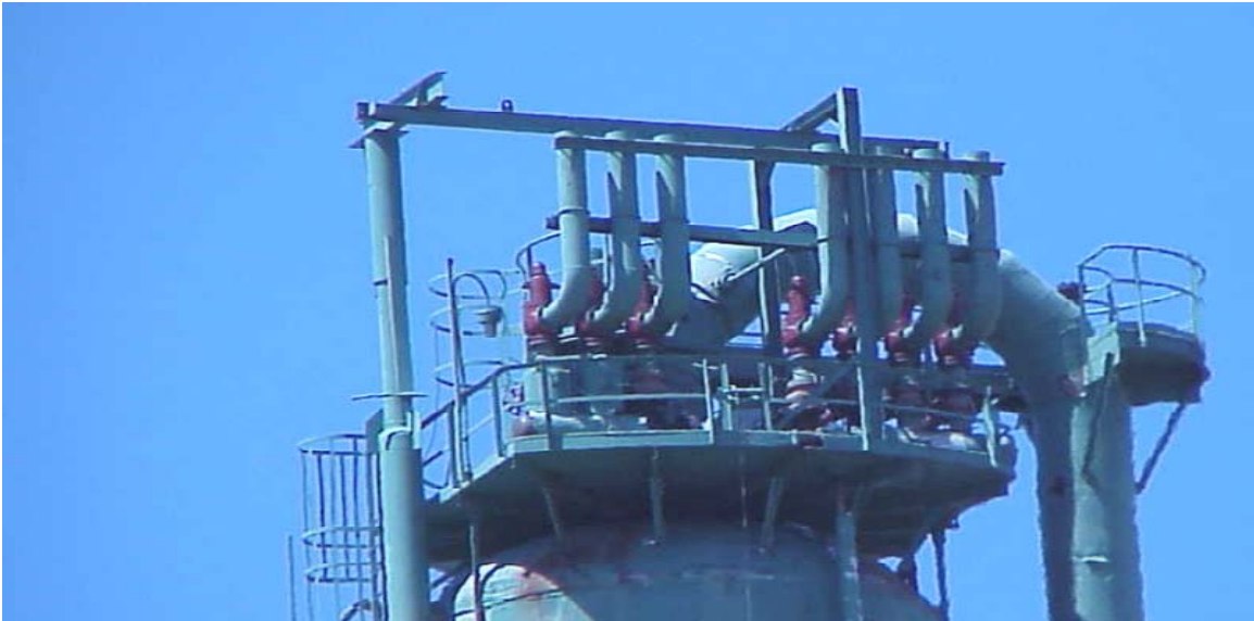
Figure 2.2 Seven 6" Diameter Pressure Relief Devices and Exhaust "Horns" Valero Refinery
