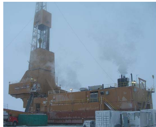
Figure 5: Doyon 14 rig and pipeshed, February 2007, during early operations on Mount Elbert-01, ANS MPU
