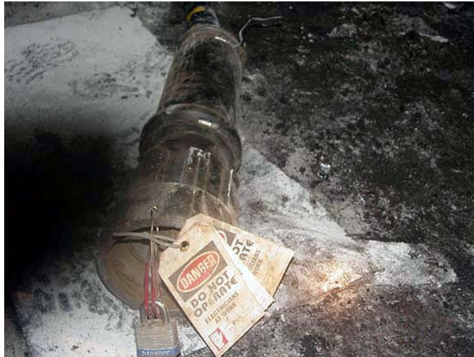
A photo of a properly locked and tagged equipment plug.
