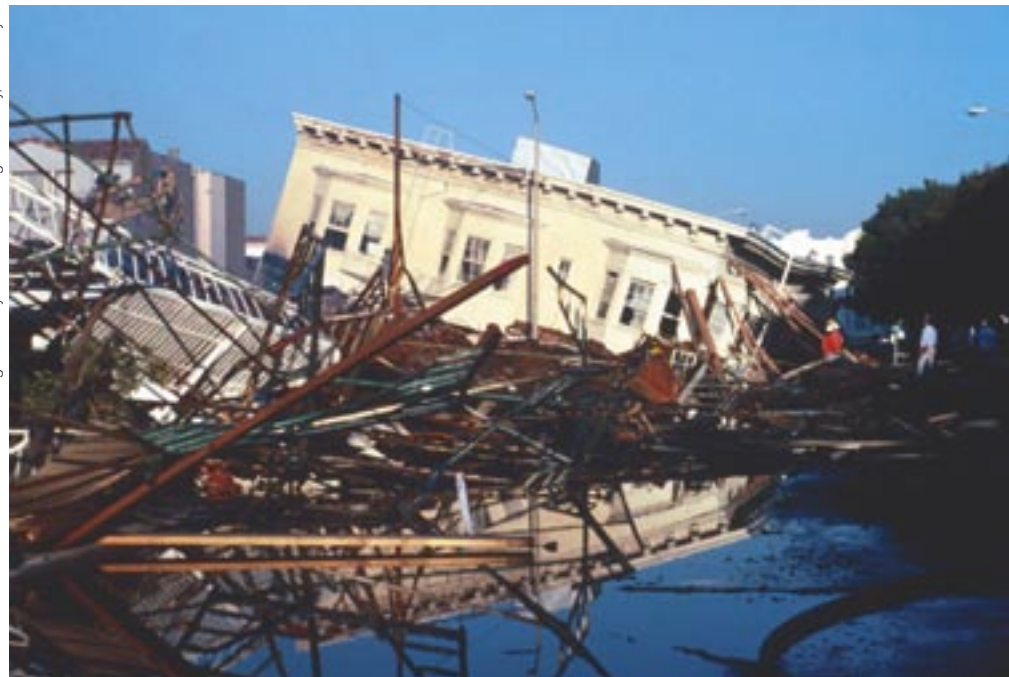
Collapsed and burned buildings shown at Beach and Divisadero streets in the Marina District, San Francisco.
