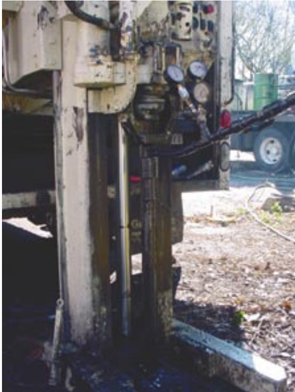
Weston Solutions, Inc.'s Emulsified Zero-Valent Iron remediation technology in process at a client site.
