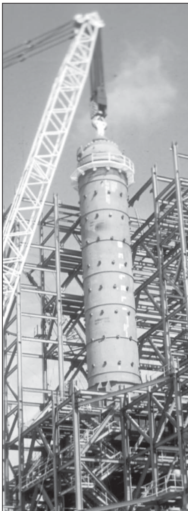
Radiant syngas cooler installation
