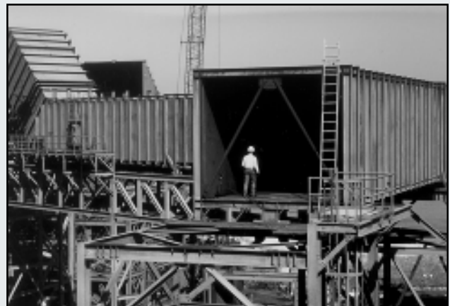
Worker inspecting ductwork
