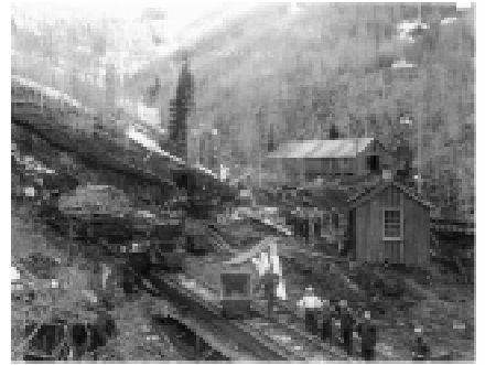
The devastation after the explosion outside on Mine No. 4, where the explosion originated
