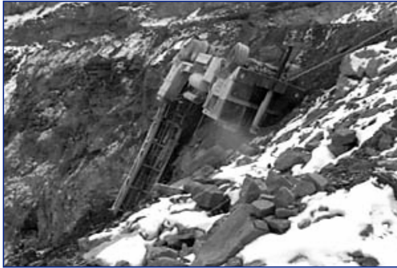
Accident No. 1: A drill toppled over a highwall, crushing the driller, when the support jack near the edge of the highwall sank into soft, unconsolidated material as the tower was being raised.
