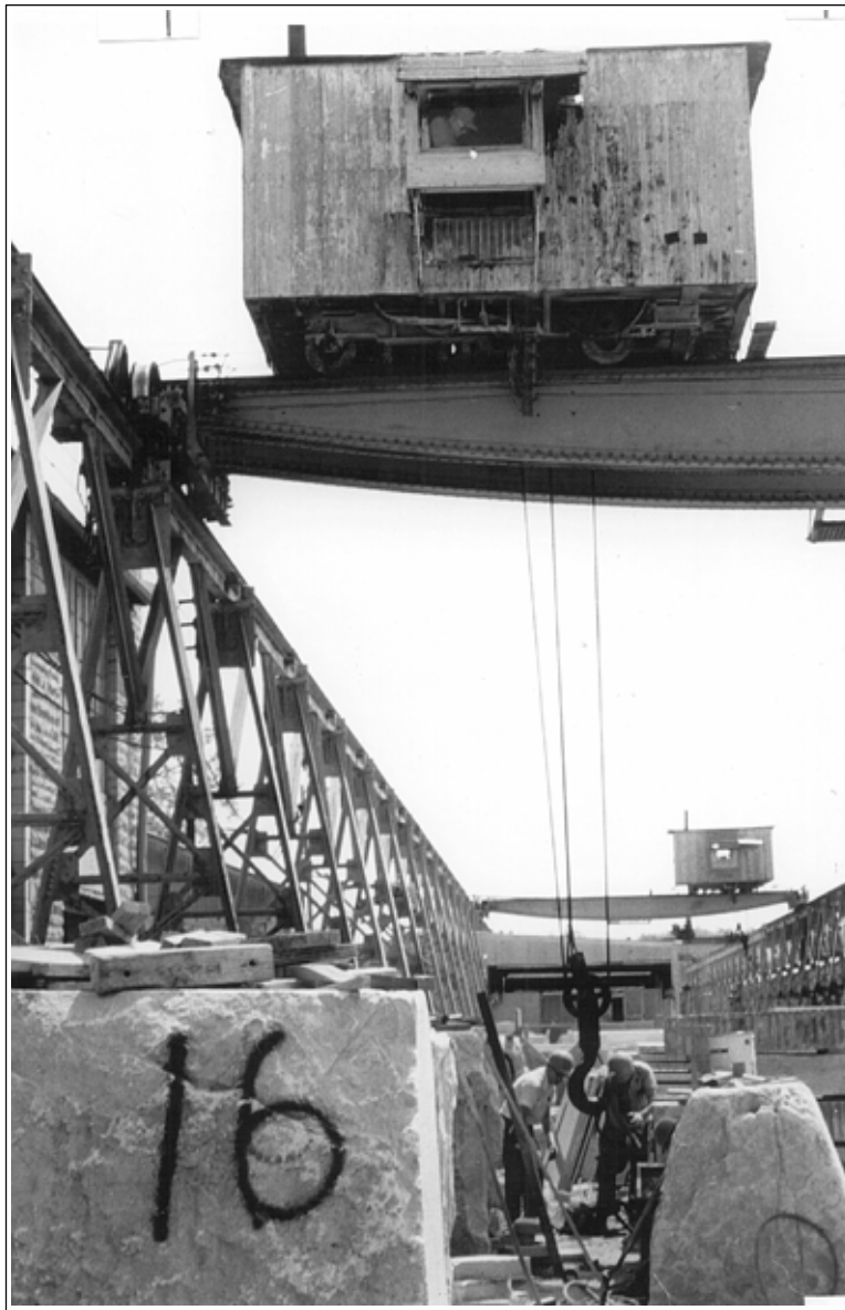
Numbered granite blocks being outfitted with a sling prior to movement to a transportation area.
