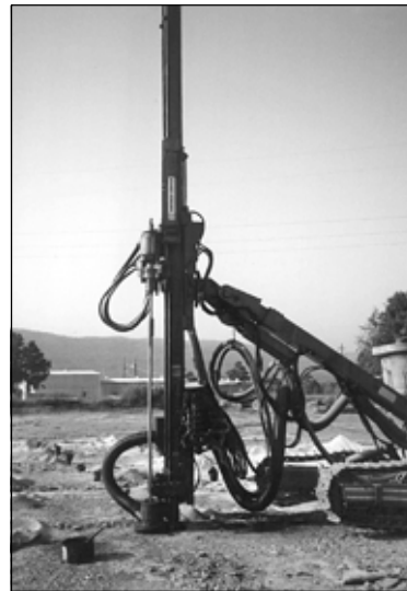
Gardner-Denver track drill with dust collector at drill collar.
