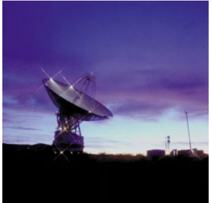
The Goldstone Deep Space Communications Complex, located in California’s Mojave Desert, is one of three complexes in NASA’s Deep Space Network (DSN).
