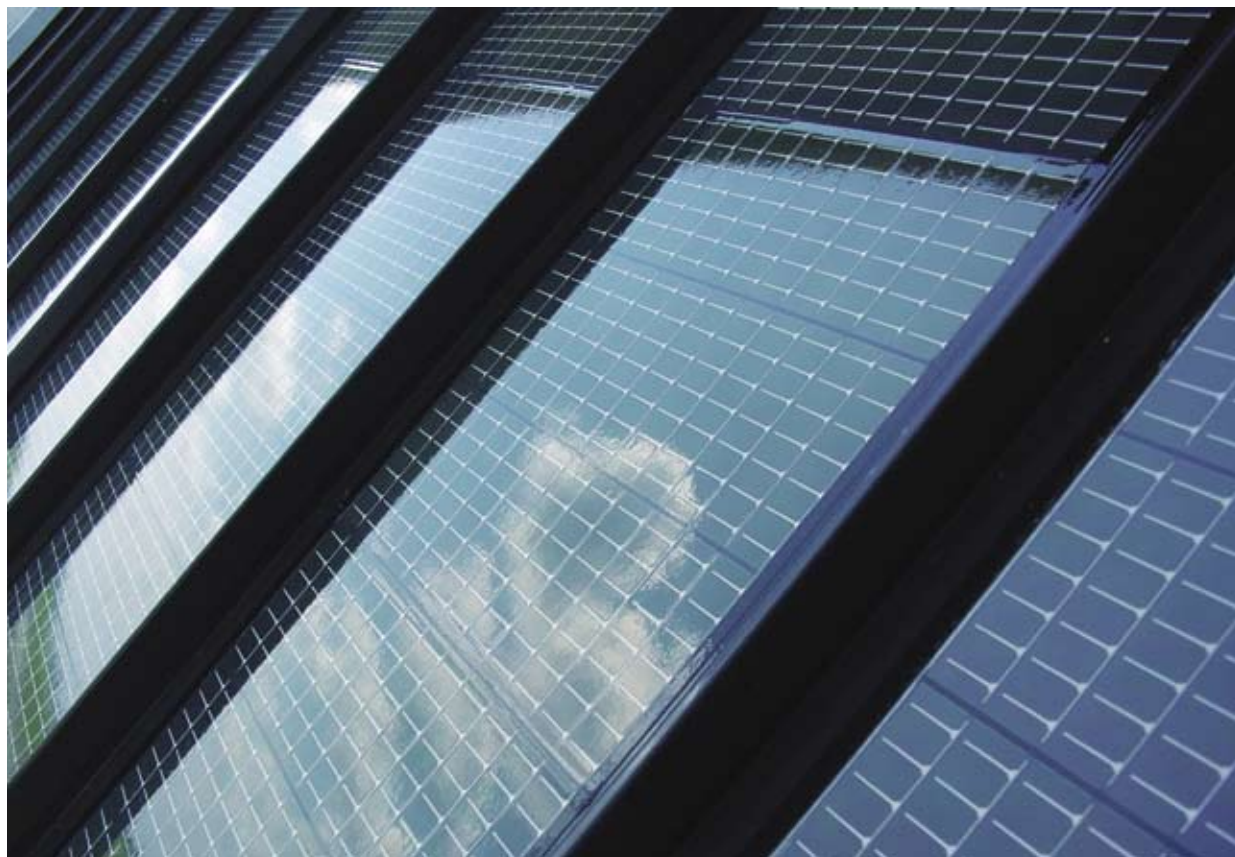
Thin film solar cells derived from amorphous silicon, pictured here, are gaining more and more attention in a market otherwise dominated by mono- and poly-crystalline silicon solar cells.
