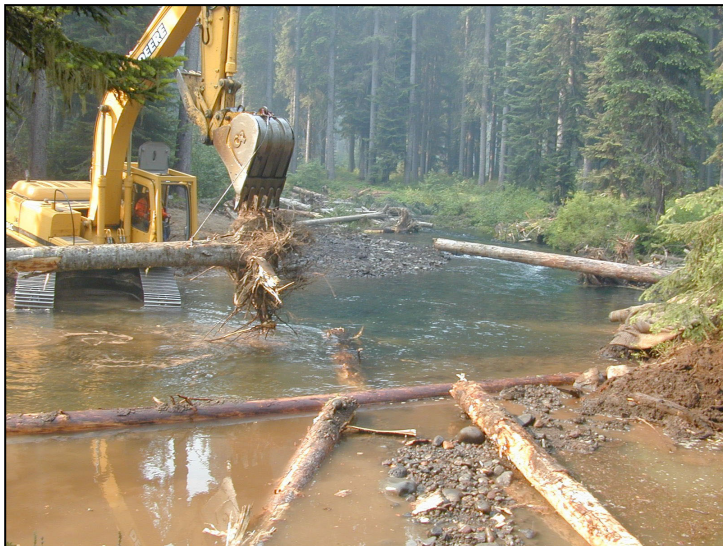
Photo 3 - Restoration activities in the Deschutes Province included log placement in the stream for the enhancement of bull trout spawning habitat.
