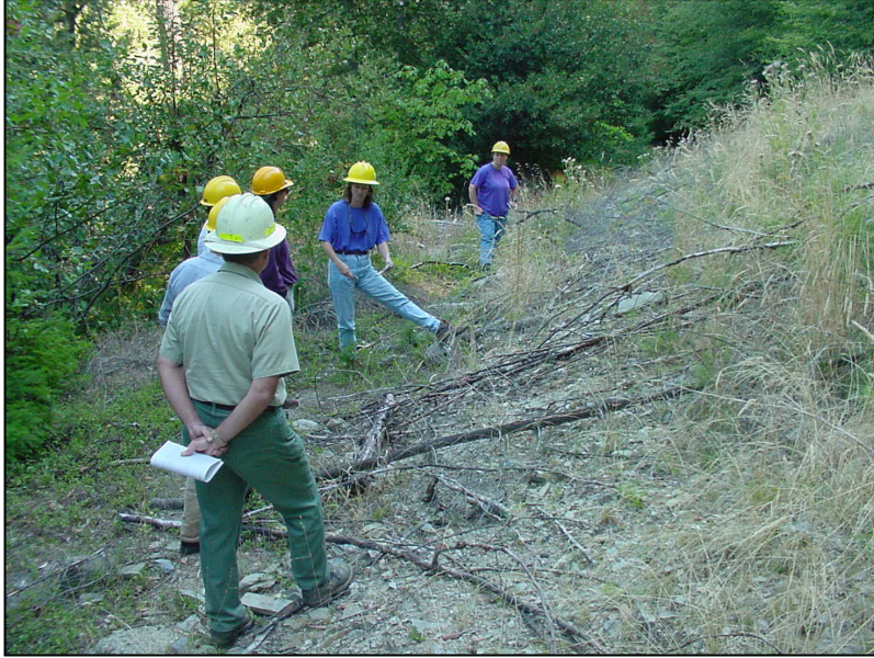
Photo 1 - The methods and objectives of road decommissioning are presented to the Klamath Provincial Advisory Committee during the watershed monitoring review.
