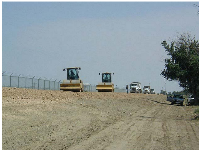
USIBWC at work on El Paso levee
