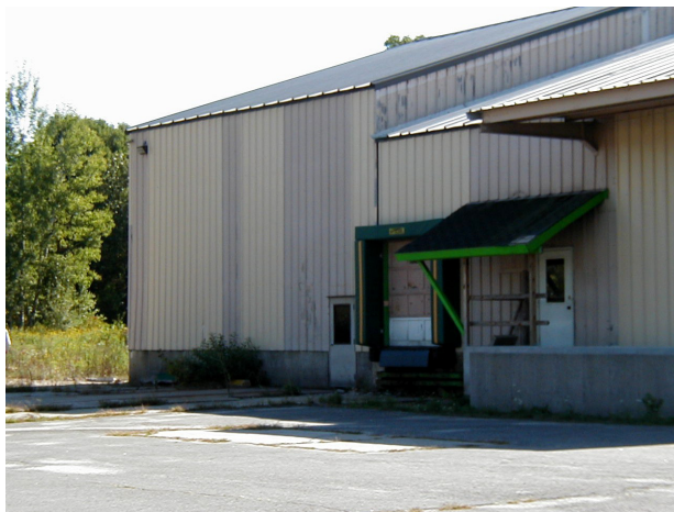
Former vermiculite processing facility in Easthampton.
