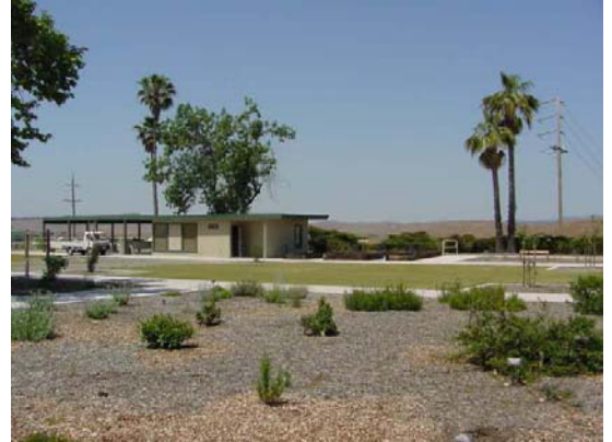
Future site of the Friant Water Education Center
