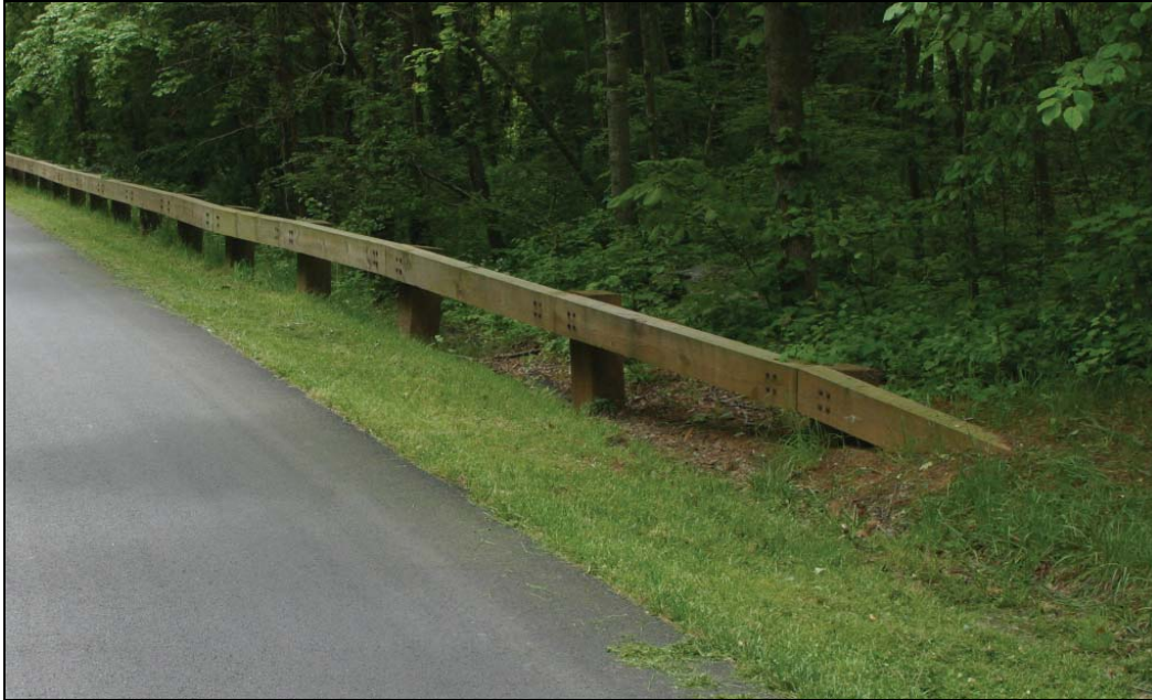
Figure 3.20: Steel-Backed Timber Buried in Backslope
