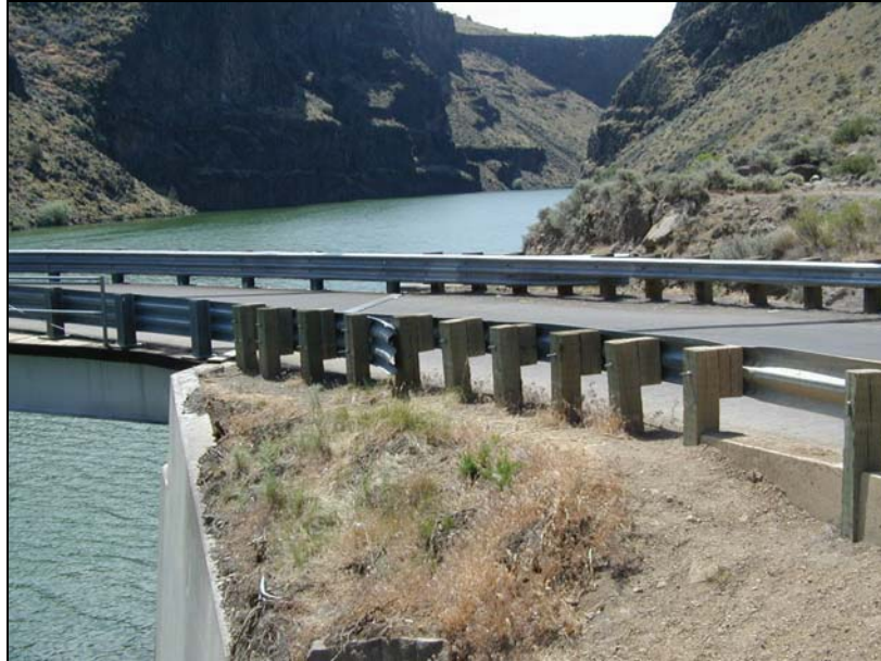
Figure 3.21: W-Beam Transition
