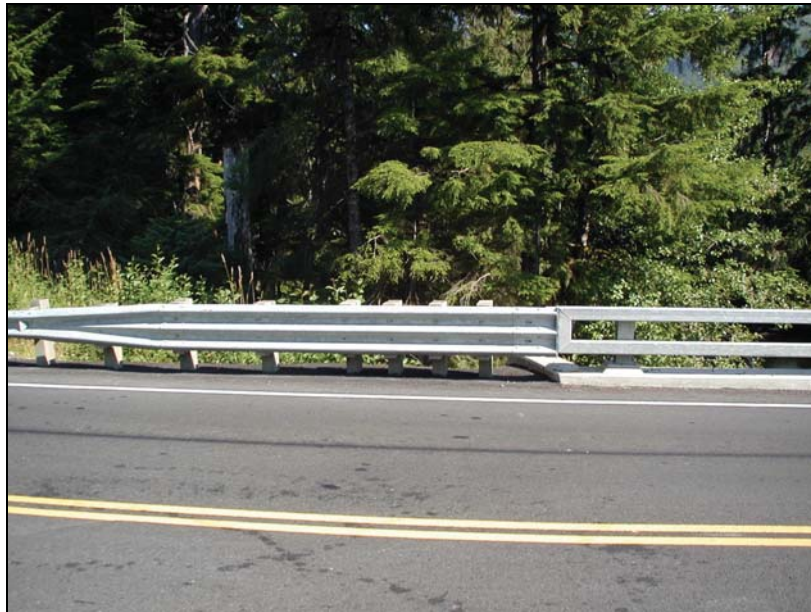
Figure 3.22: W-Beam to Thrie-Beam Transition
