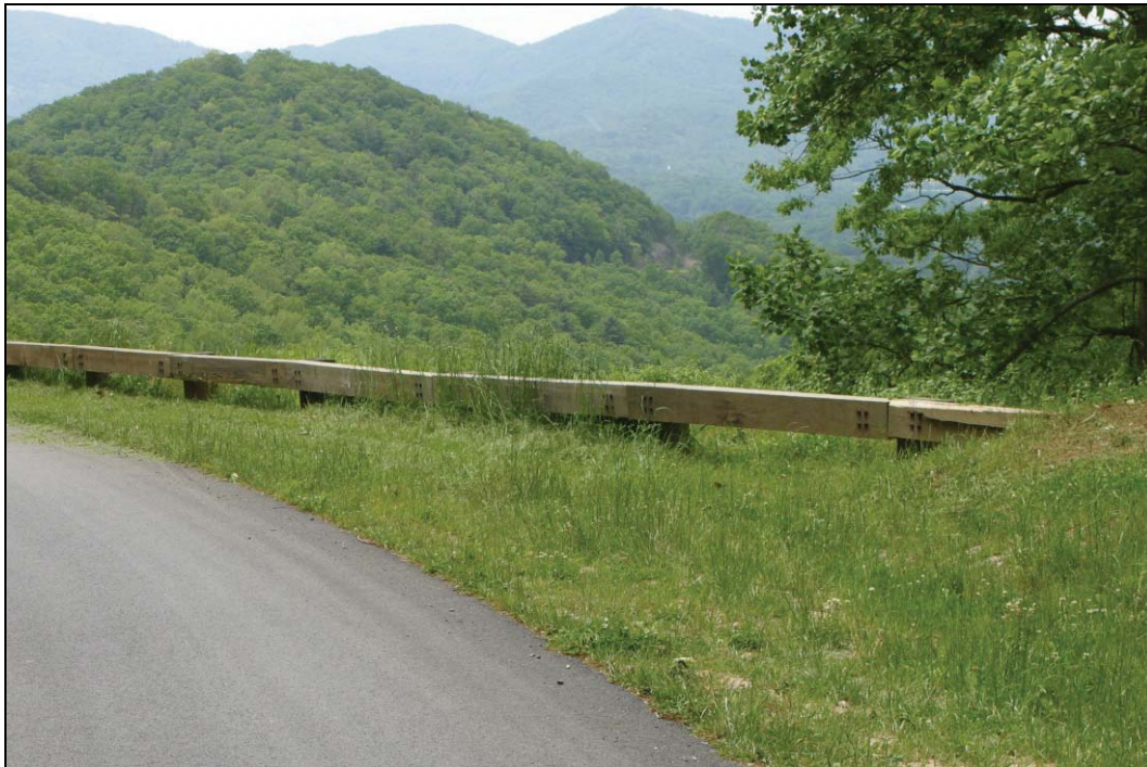
Figure 3.20: Steel-Backed Timber Buried in Backslope
