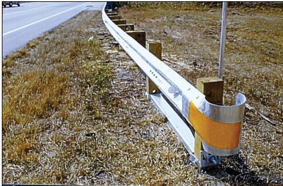
Figure 3.16: W-Beam Flared End
