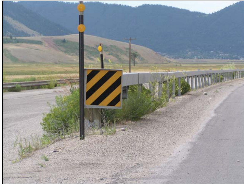
Figure 3.14: W-Beam with MELT
