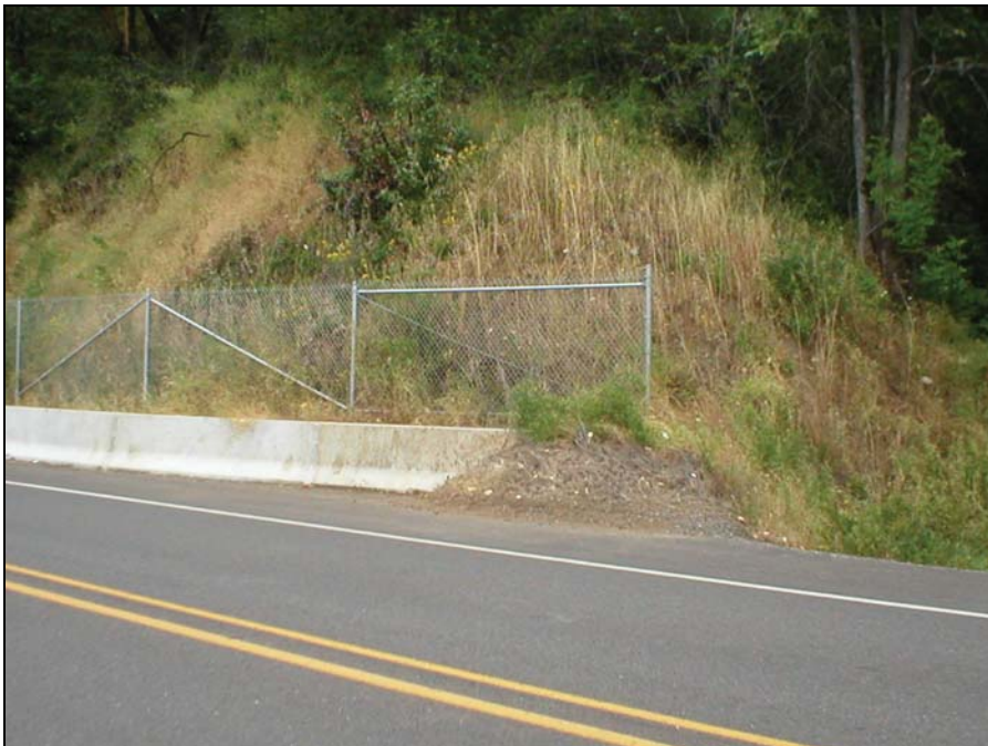
Figure 3.18: Concrete Safety Shape Buried in Backslope
