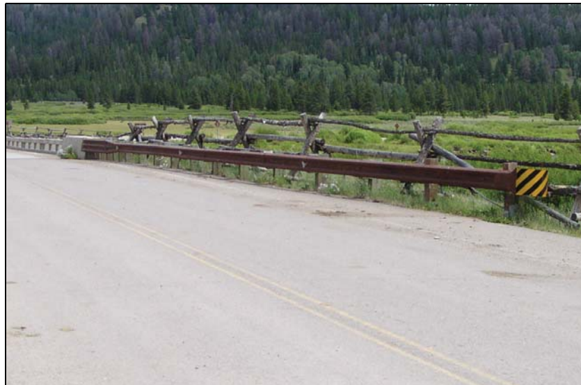
Figure 3.14: W-Beam with MELT
